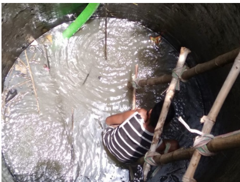
Laborers stated cleaning process
