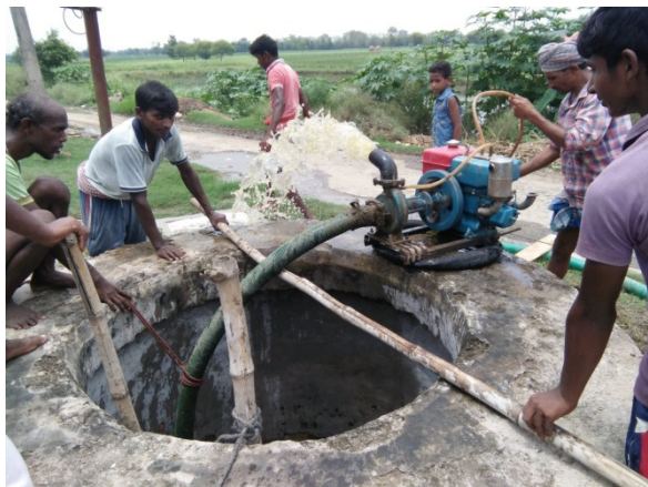
Dewatering of Well
