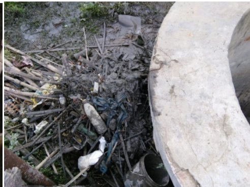
Waste material removed from well
